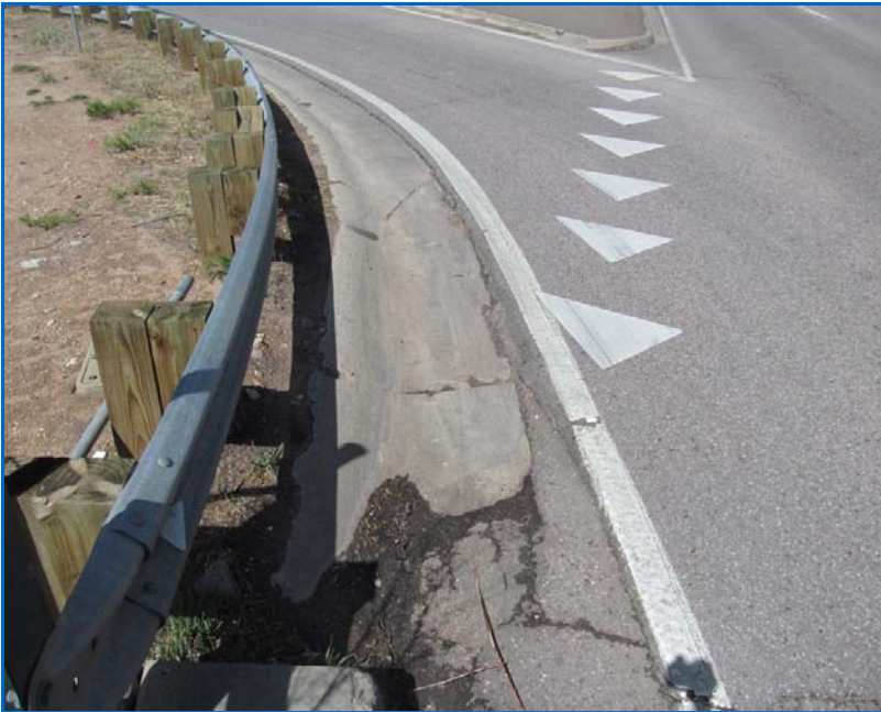
CSG-F.85-08.23 Settled and cracked curb and gutter at southwest.JPG
