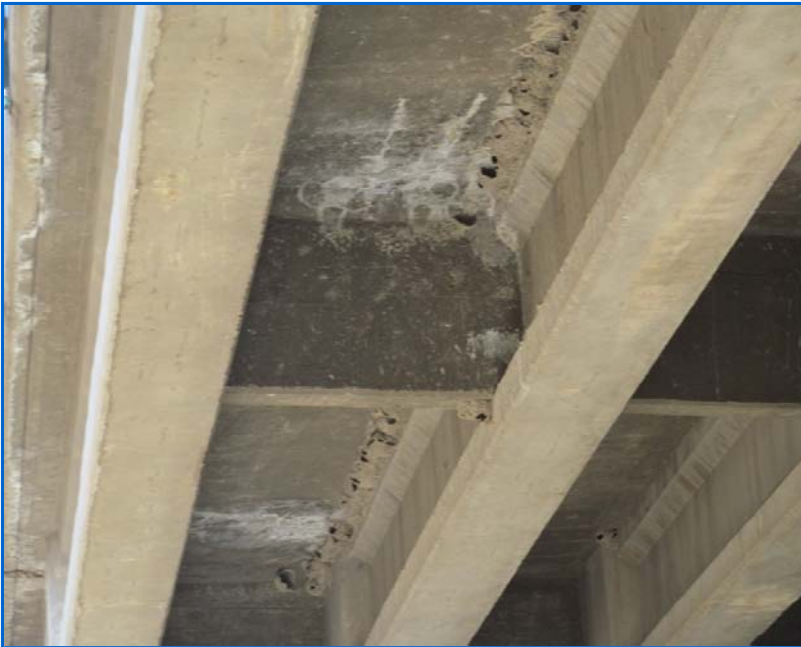
CSG-F.85-08.23 Cracks with efflorescence in soffit in Span 4.JPG
