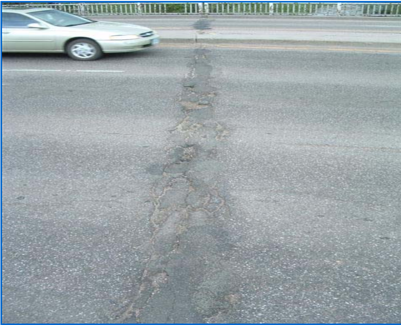
CSG-F.85-08.23 JOINT CONDITION ABOVE PIER 4.JPG
