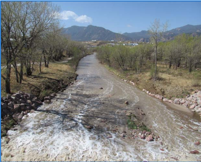
CSG-F.85-08.23 Channel looking downstream.JPG
